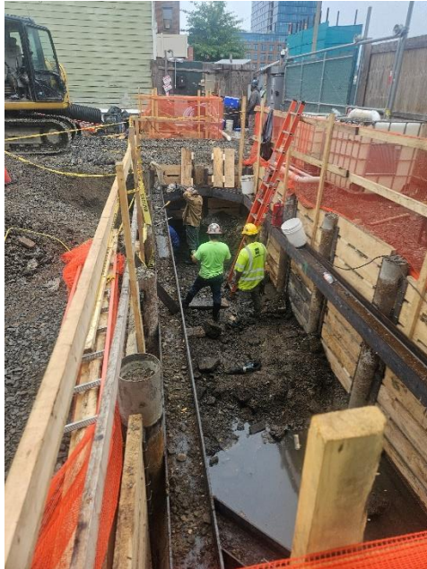
Photo 1: View of contractor welding I-beams to pilings, facing West.
