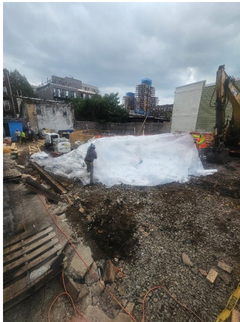
Photo 2: View of contractor covering stockpile with odor control foam and poly sheeting, facing Southwest.
