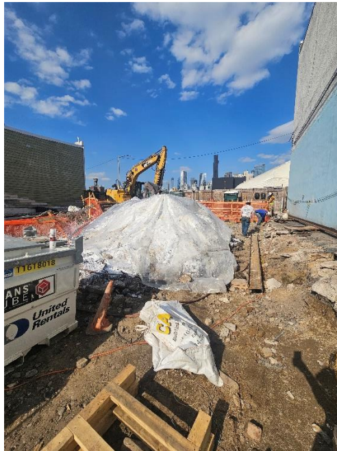
Photo 2: View of contractor covering stockpile with odor control foam and poly sheeting, facing North.
