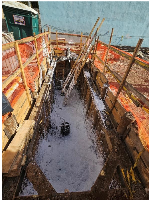
Photo 2: View of piling excavation covered with odor suppressant foam, facing East.
