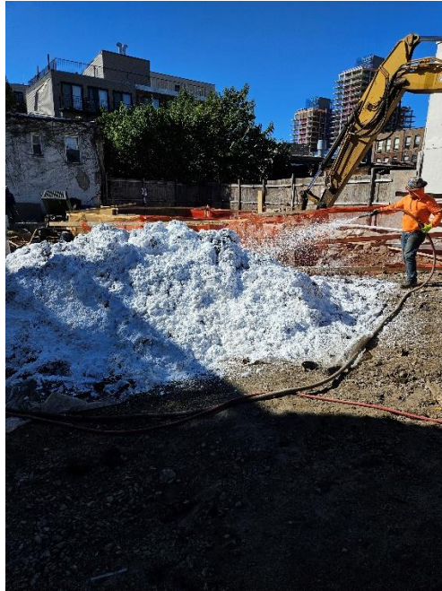
Photo 2: View of stockpile covered with odor suppressant foam, facing Southwest.
