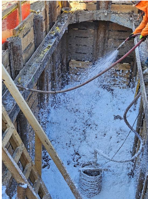
Photo 1: View of concurrent odor suppressant foam application during excavation, facing West.
