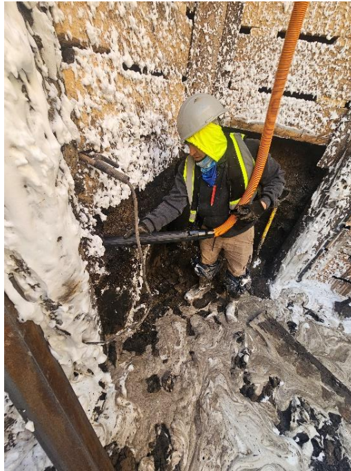
Photo 1: View of contractor using shop vac to remove observed product, facing Southwest.
