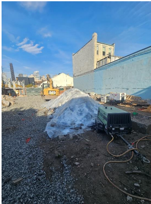
Photo 2: View of soil stockpiles covered with odor suppressant foam and poly sheeting, facing Northeast.
