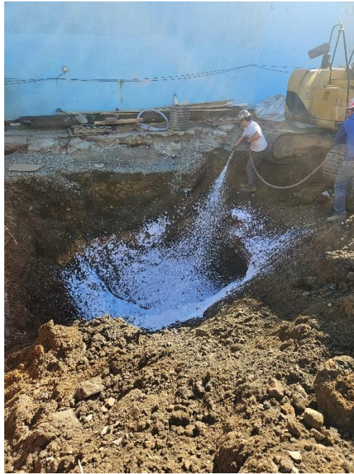
Photo 1: View of contractor applying odor suppressant foam during excavation, facing East.
