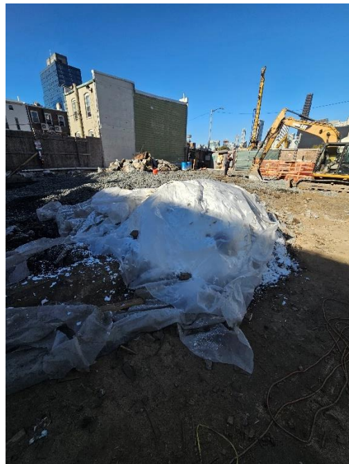
Photo 2: View of soil stockpiles covered with odor suppressant foam and poly sheeting, facing Northwest.
