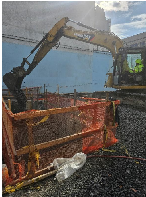
Photo 2: View of contractor backfilling CS02/CS03 excavation, facing Southeast.
