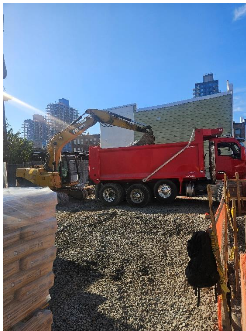
Photo 2: View of contractor loading C&D for off-Site disposal, facing West.
