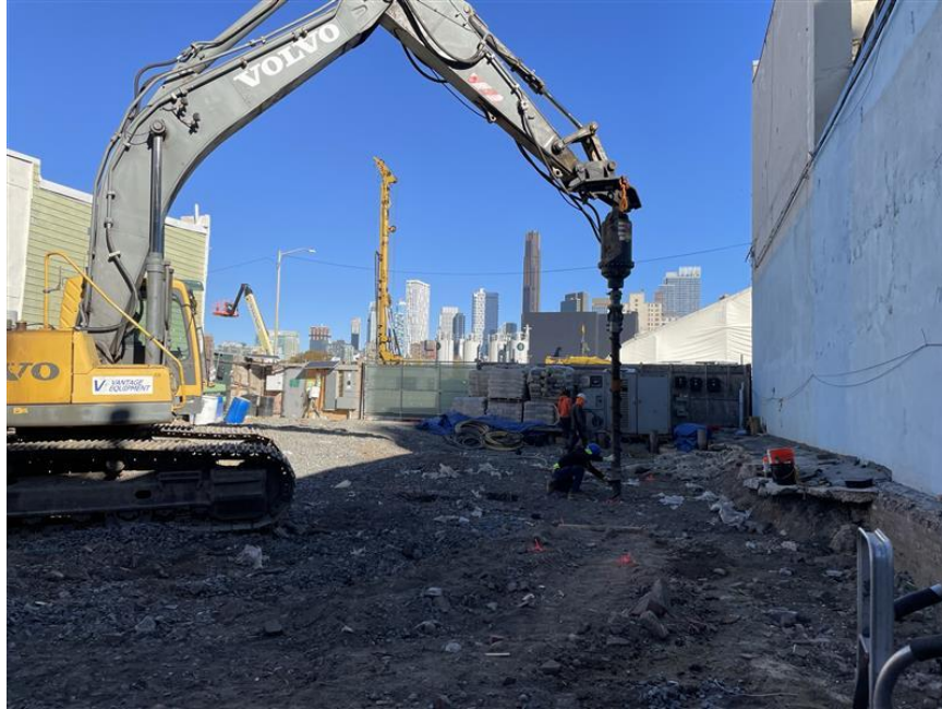
Photo 1: View of contractor installing structural piles, facing Northeast.
