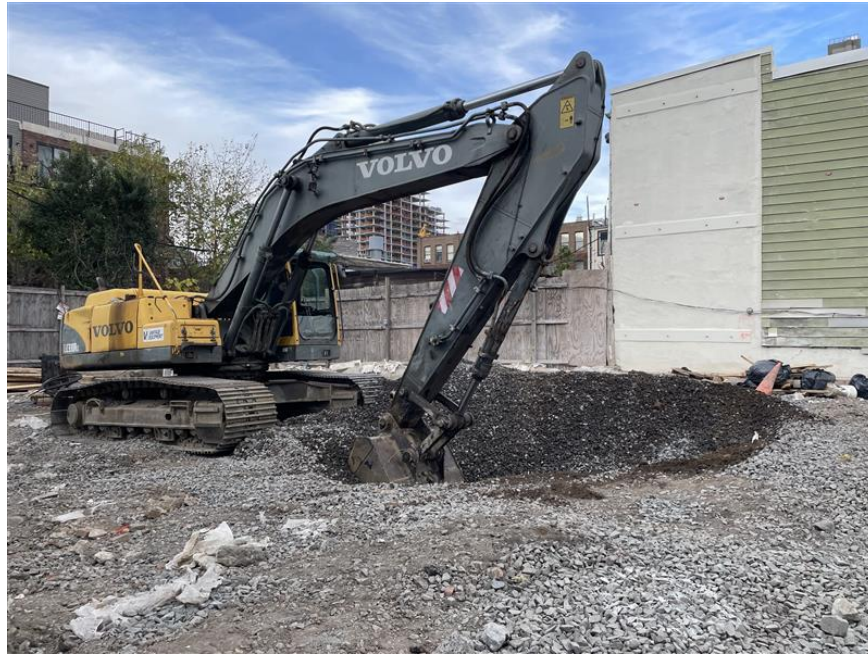
Photo 1: View of contractor excavating for soil samples, facing Southwest.
