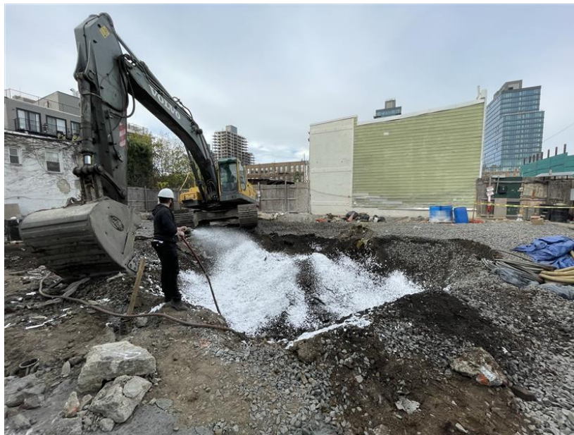
Photo 2: View of contractor spraying odor suppressant in excavation, facing Southwest.
