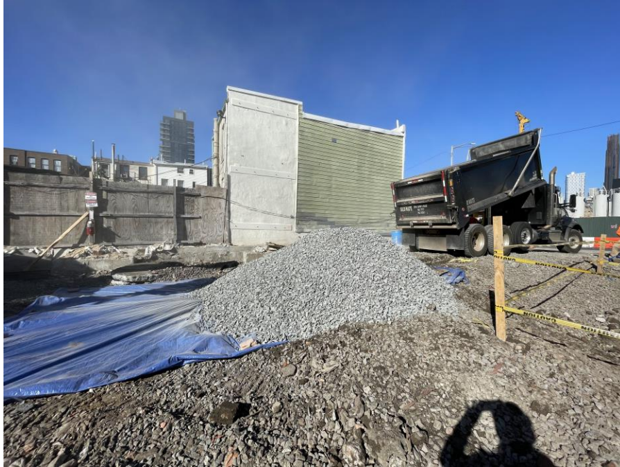
Photo 1: View of contractor stockpiling imported clean gravel, facing Northwest.
