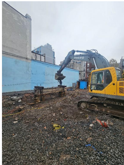
Photo 2: View of contractor constructing test pile apparatus, facing Southeast.
