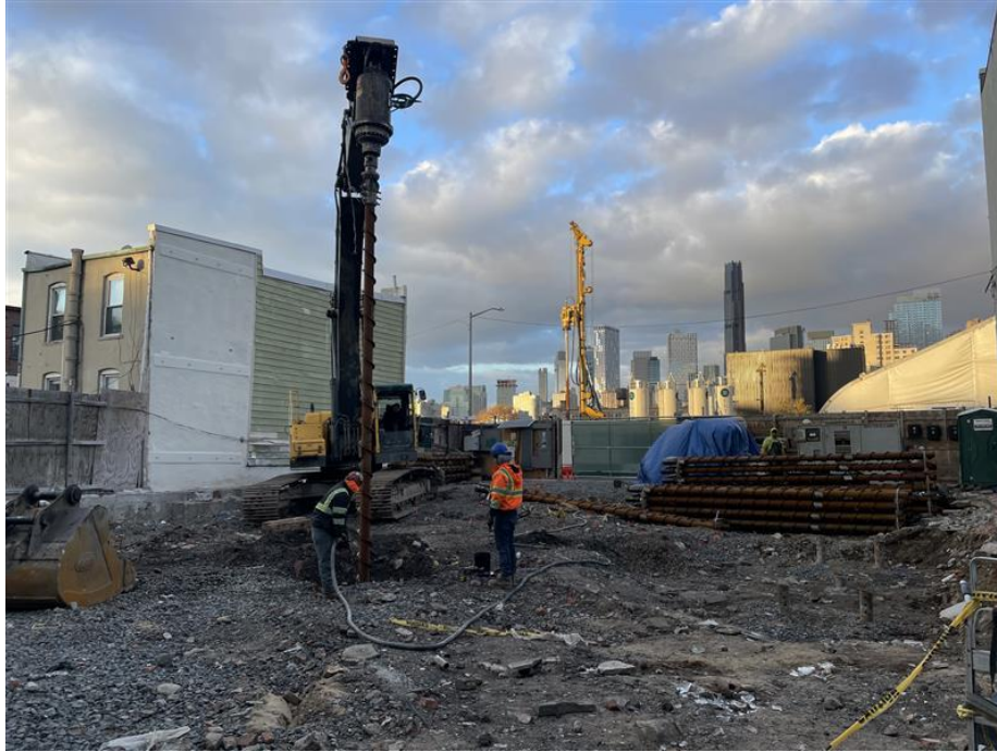
Photo 1: View of Blanco installing structural pile, facing Northeast.
