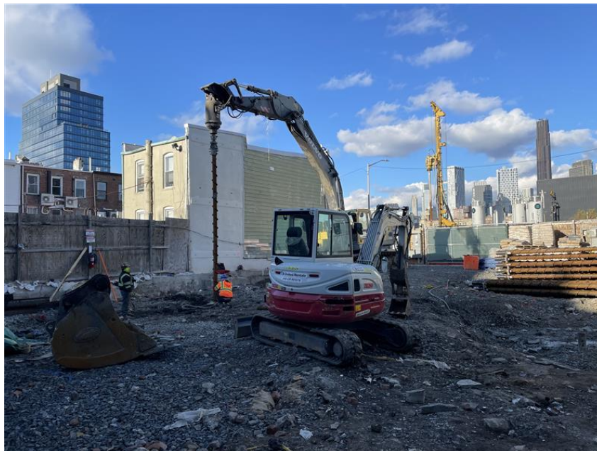
Photo 2: View of Blanco installing structural pile, facing Northeast.
