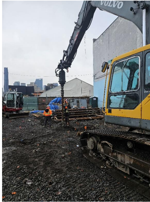
Photo 1: View of Blanco installing structural pile, facing North.
