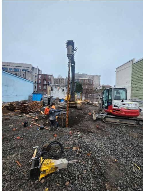
Photo 1: View of Blanco installing structural pile, facing South.
