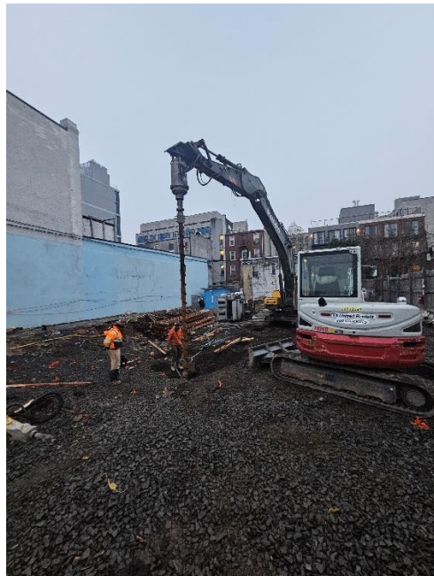
Photo 2: View of Blanco installing structural pile, facing Southeast.
