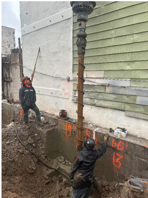
Photo 2: View of Blanco installing structural pile, facing Southwest.
