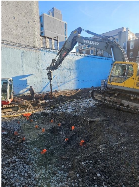
Photo 1: View of Blanco installing structural pile, facing Southeast.
