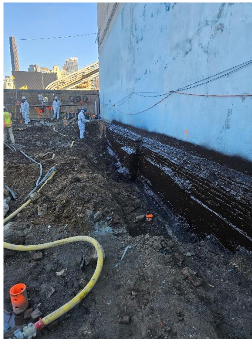
Photo 2: View of A1 applying waterproofing to East boundary foundation wall, facing North.
