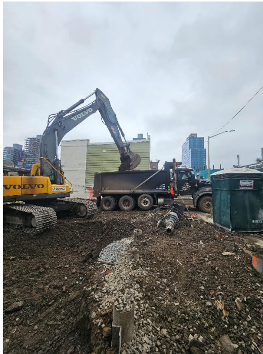
Photo 2: View of contractor loading soil for off-Site disposal, facing West.
