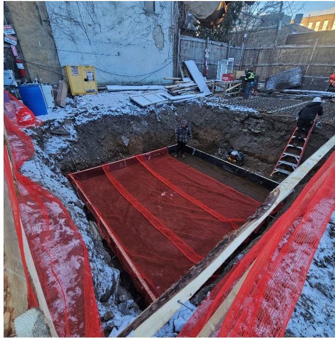
Photo 1: View of contractor laying red snow fencing as a demarcation barrier, facing Southwest.
