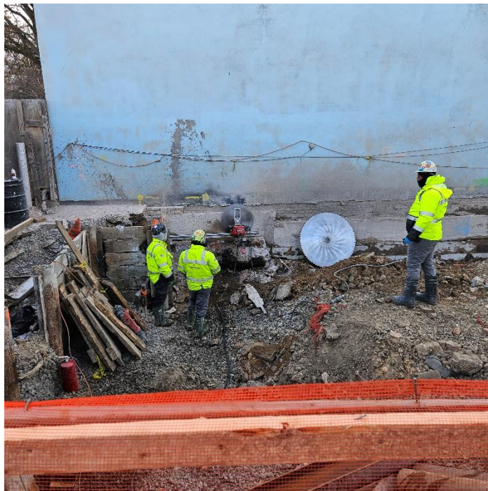
Photo 2: View of contractor saw cutting adjoining building footings, facing East.
