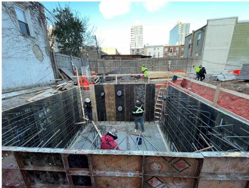
Photo 2: View of contractor installing foundation wall frames, facing West.
