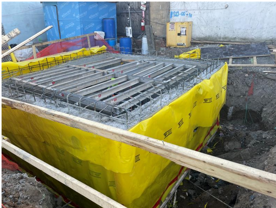
Photo 2: View of contractor installing vapor barrier to the water tank, facing southeast.
