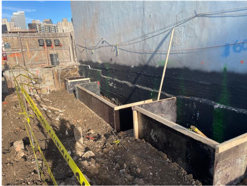
Photo 1: View of prepped footing frames, facing Northeast.
