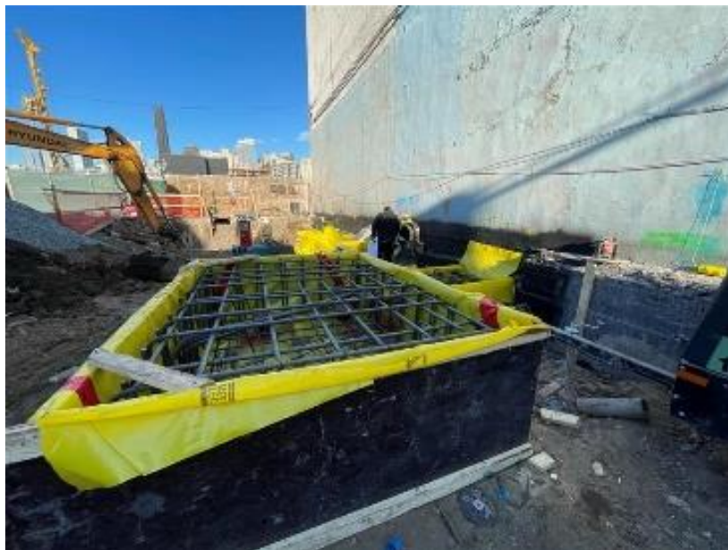
Photo 2: View of contractor installing rebar in footing frames, facing northeast.
