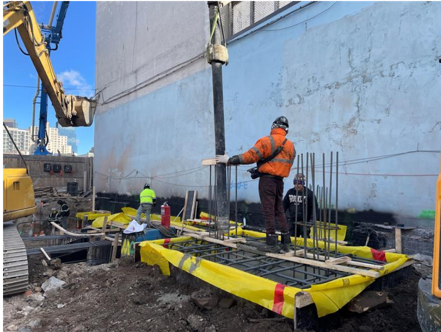
Photo 1: View of contractor pouring concrete into footing frames, facing Northeast.
