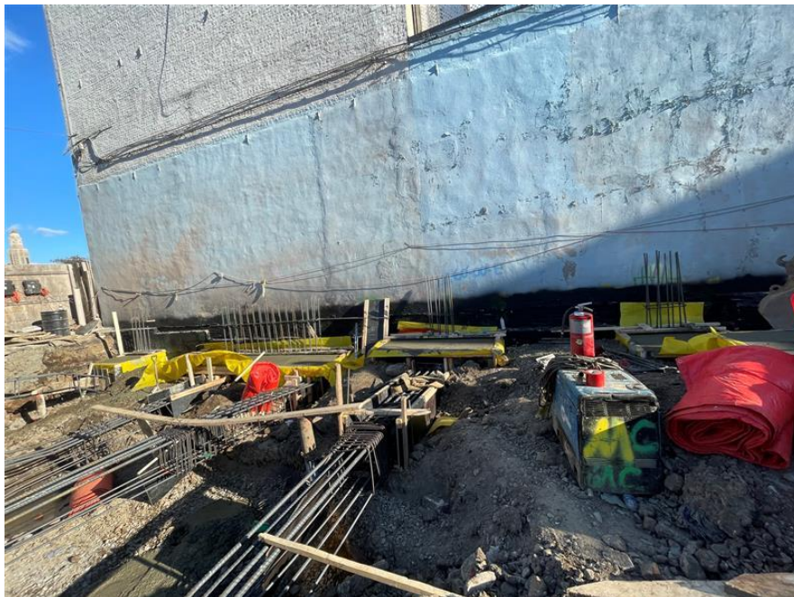
Photo 2: View of completed footing frames, facing East.
