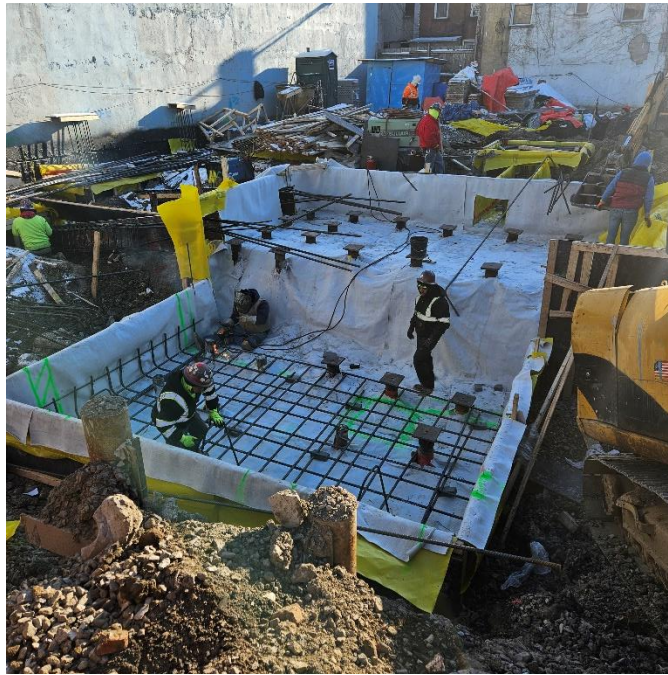
Photo 1: View of contractor installing rebar for footing forms, facing Southeast.
