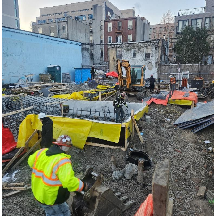
Photo 1: View of contractor installing rebar in footing forms, facing Southeast.
