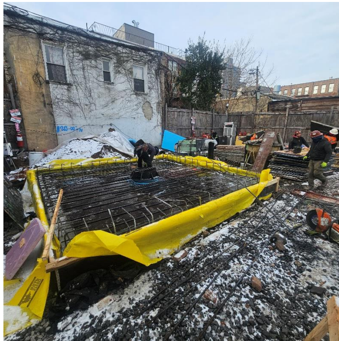
Photo 2: View of contractor installing rebar for water tank, facing Southwest.
