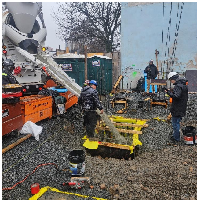
Photo 2: View of contractor pouring concrete for footing, facing East.
