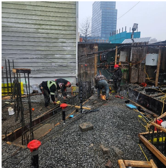
Photo 2: View of contractor installing rebar for foundation, facing Northwest.
