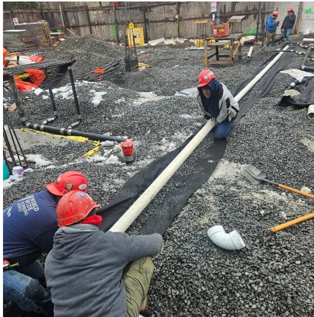
Photo 1: View of contractor installing SSDS piping, facing Southwest.
