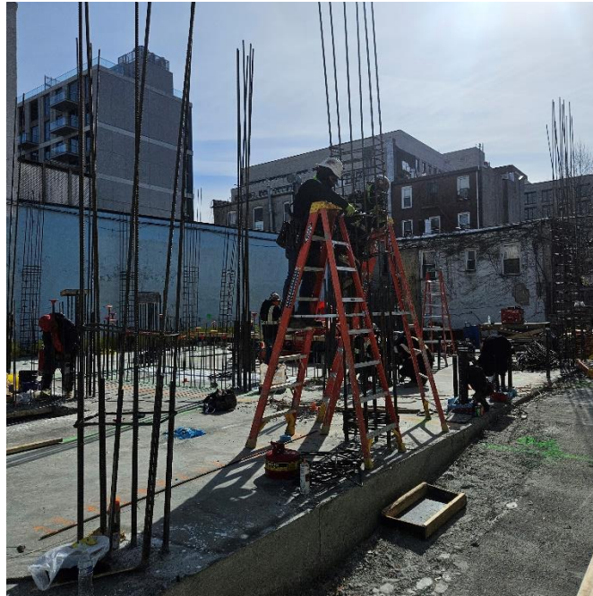
Photo 1: View of contractor installing rebar for superstructure, facing Southeast.
