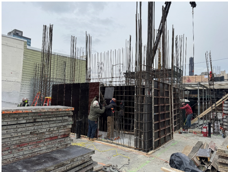
Photo 2: View of contractor installing rebar for superstructure, facing Northwest.
