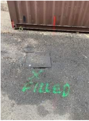
Picture 1 FILLED STORM DRAIN.
