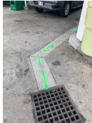
Picture 4: STORM DRAIN LINE 1-2' IN DEPTH
