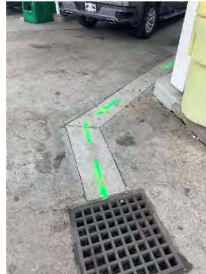
Picture 4: STORM DRAIN LINE 1-2' IN DEPTH
