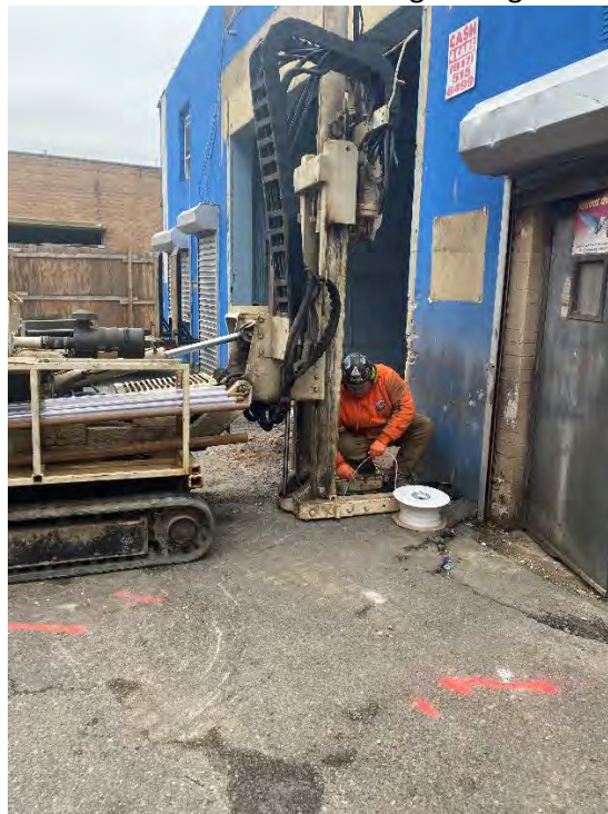
Photo 2: View of soil vapor point installation VP-05.
