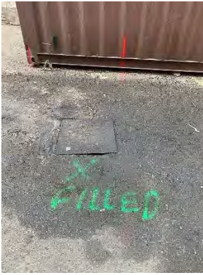
Picture 1 FILLED STORM DRAIN.
