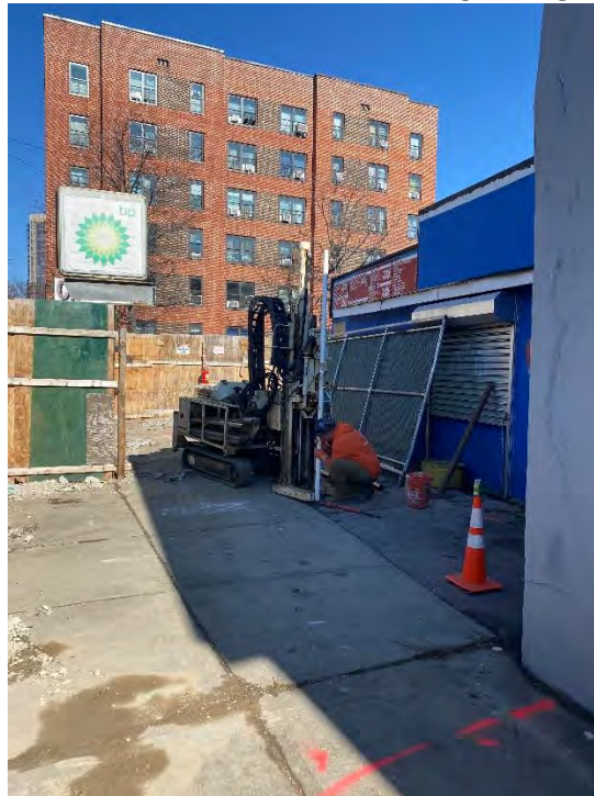
Photo 2: View of monitoring well installation MW-09.
