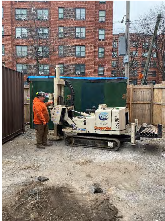
Photo 1: View of HA-09 soil boring drilling activities.
