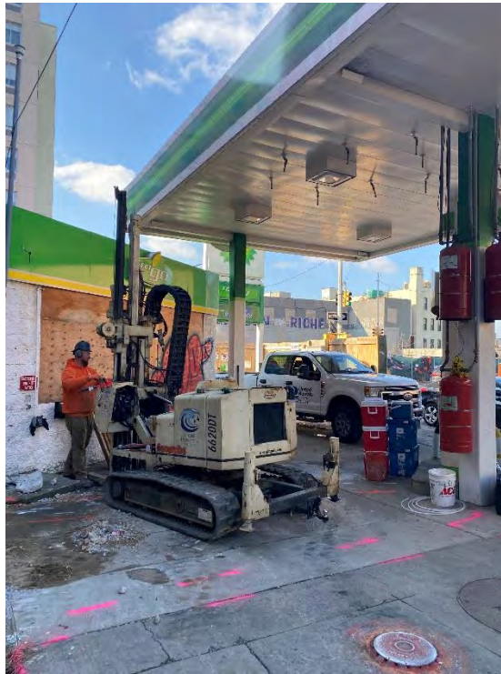
Photo 1: View of HA-02/MW-02 soil boring drilling activities.
