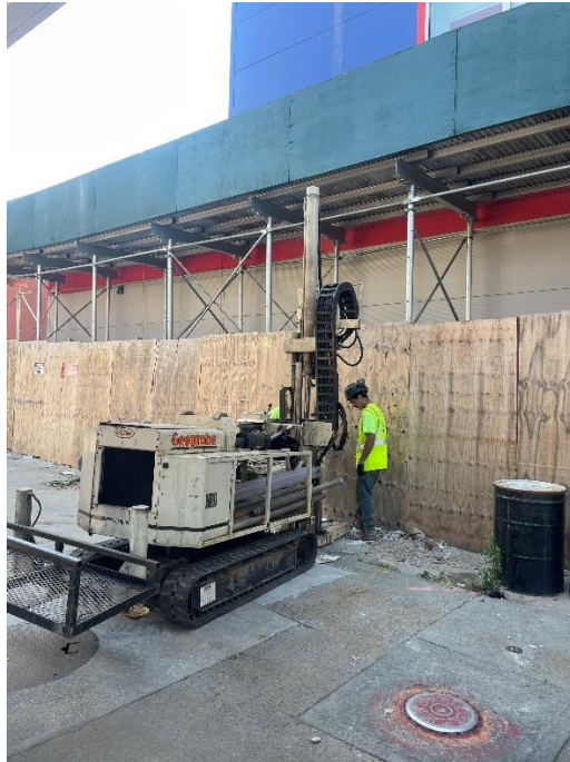
Photo 1: View of delineation boring installation, facing east.
