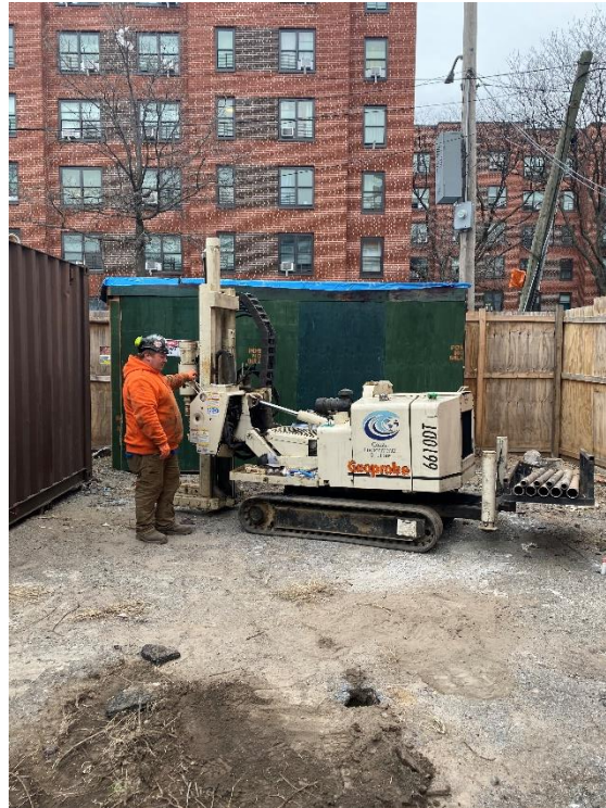
Photo 1: View of HA-09 soil boring drilling activities.
