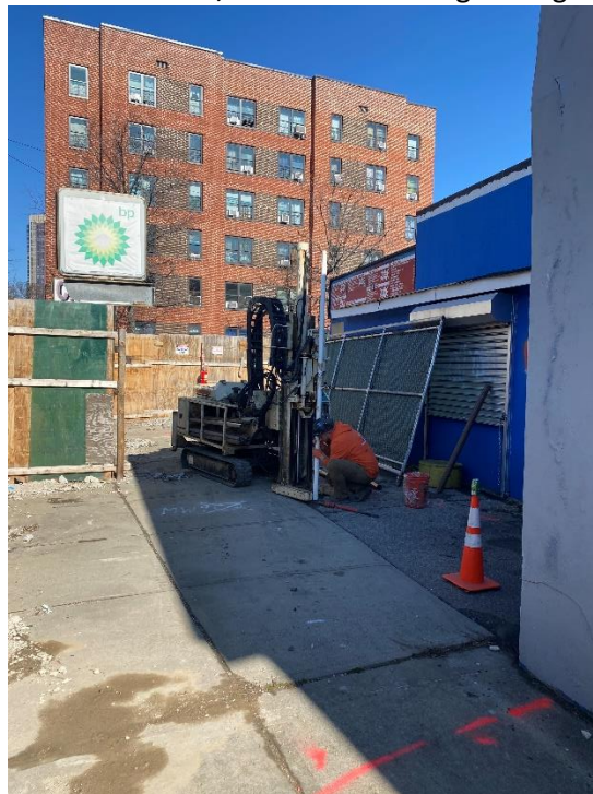
Photo 2: View of monitoring well installation MW-09.
