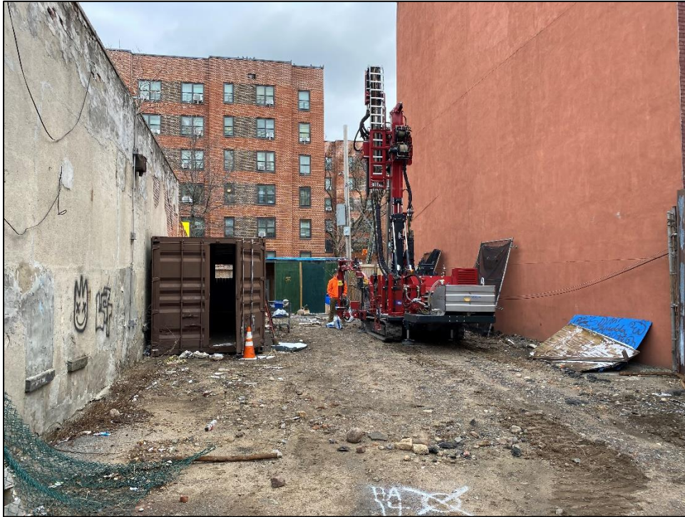
Photo 1: View of drilling activities.
