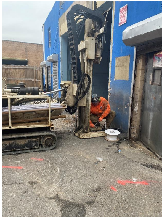
Photo 2: View of soil vapor point installation VP-05.
