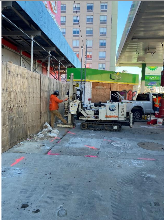
Photo 1: View of HA-26 soil boring drilling activities.
