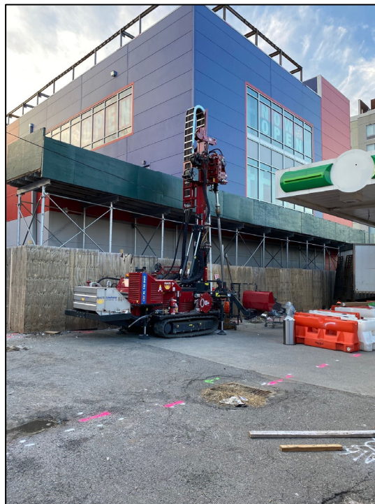
Photo 2: View of drilling activities.
