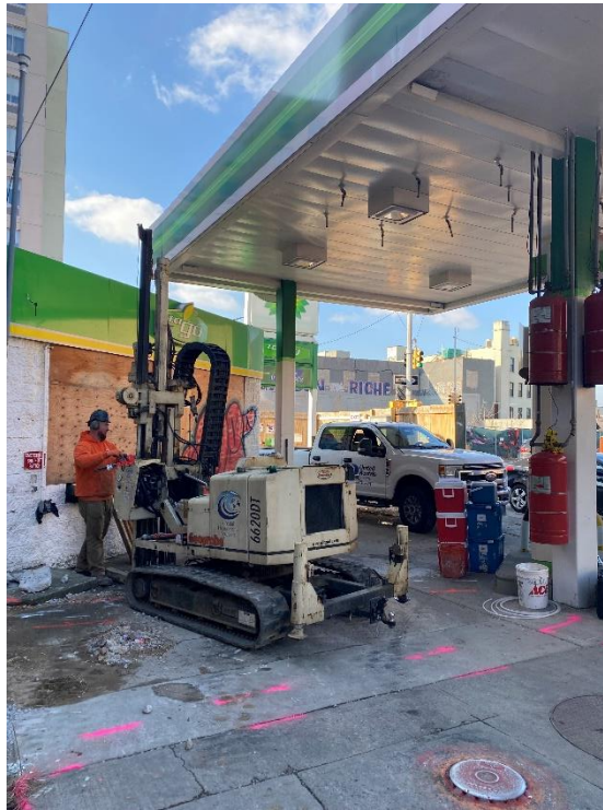
Photo 1: View of HA-02/MW-02 soil boring drilling activities.
