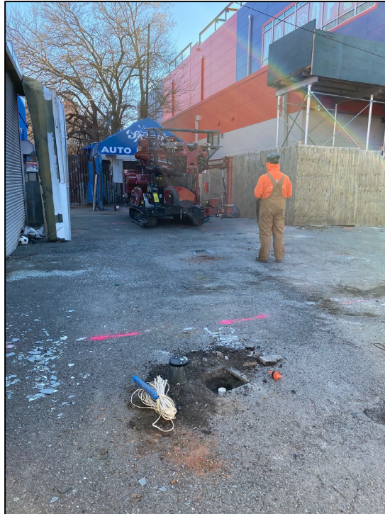
Photo 1: View of drilling activities and monitoring well installation.
