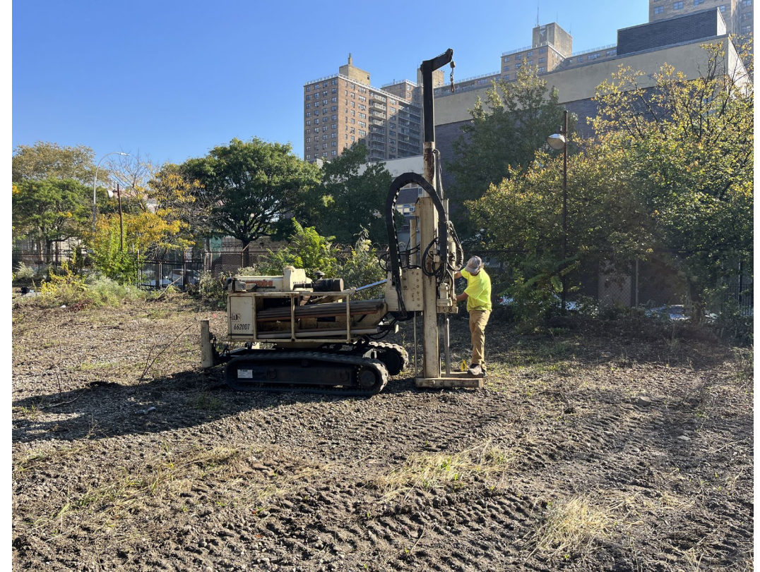
Drilling the borehole for the soil vapor implant at SV-4 location
