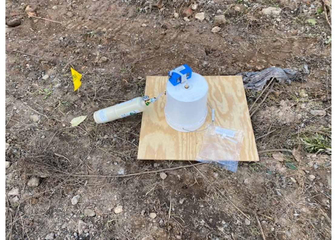
Using helium to enrich the air inside of the inverted bucket to check that there is no cross connection between the subsurface soil vapor and the outside (ambient) air.
