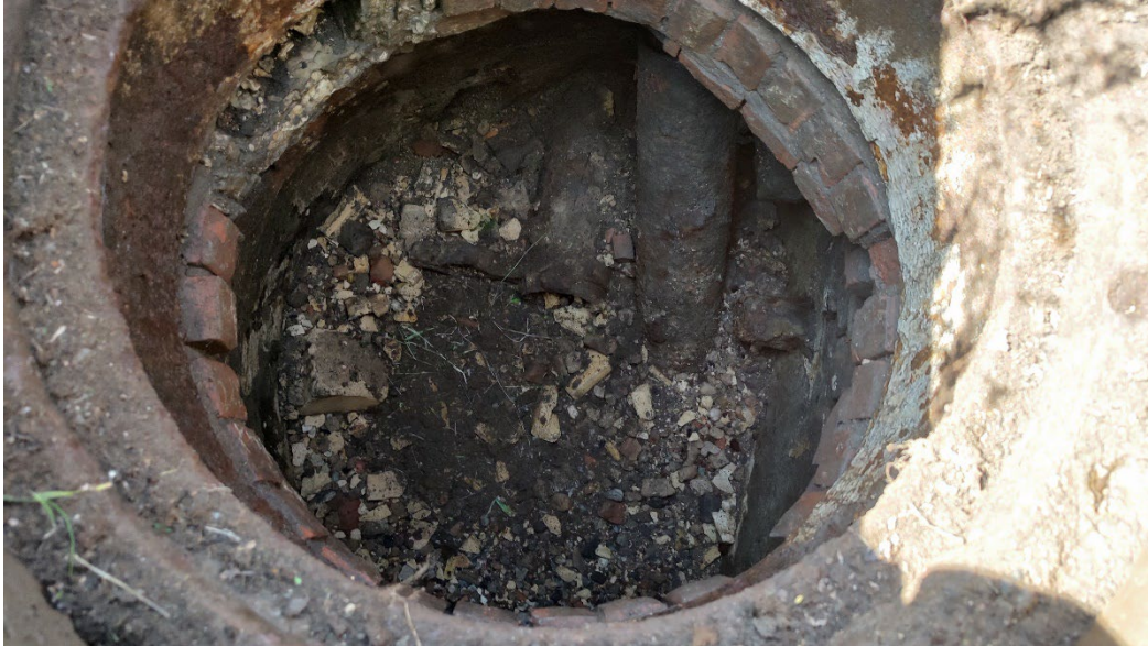
Photo 2 – View of the interior of the manhole indicated in Photo 1.
