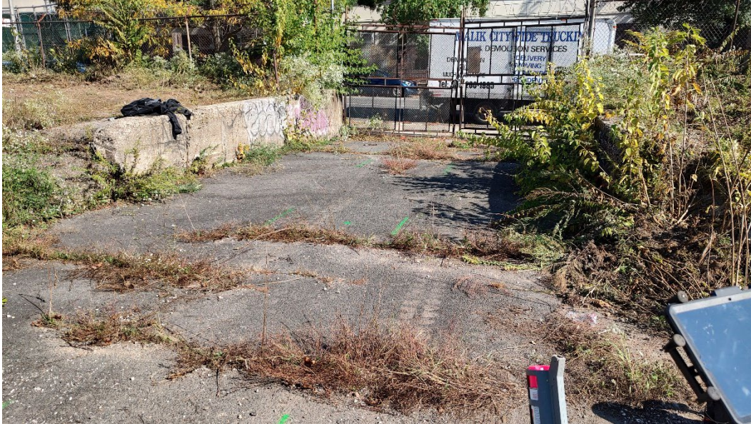
Photo 4 – View of the sanitary line at the points it was detected between the manhole pictured in Photos 1 and 2 and the central gate. An additional manhole is located immediately inside the gate, obscured in the above photo by overgrowth.
