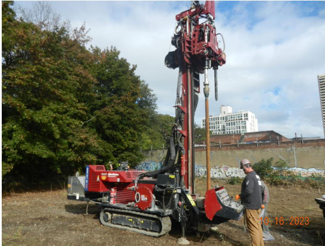
View of the Fraste Eijkelkamp Sonic Drilling rig set up on soil boring SB-7
