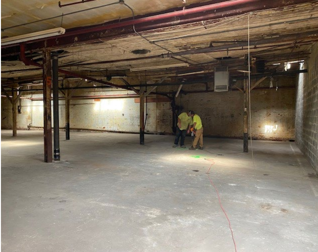
Drilling the borehole for the soil vapor implants inside 962 Franklin Avenue with a hammer drill.
