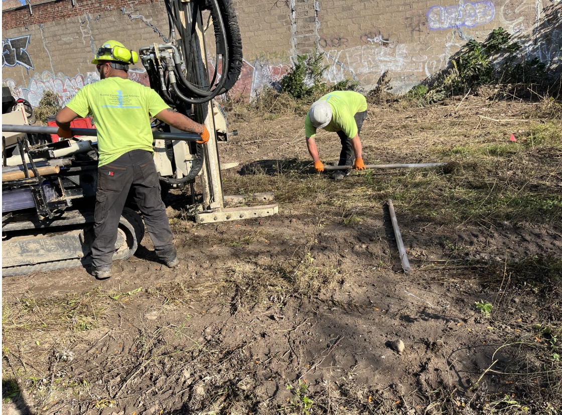
Soil sampling with the Geoprobe 7728 DT at Soil boing Location SB-1
