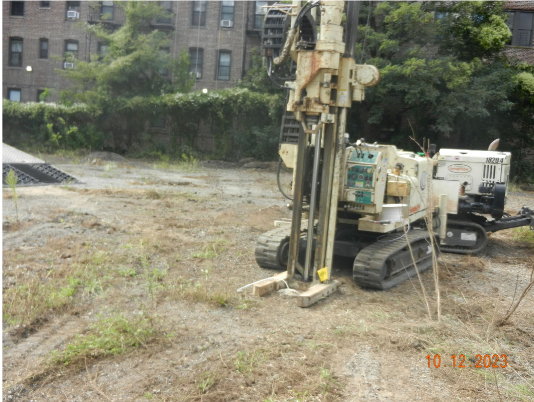
Geoprobe 7822 DT Drilling rig used for soil sampling & installing the soil vapor points
