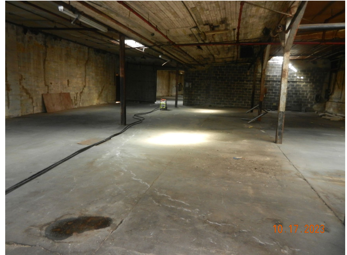
View of the interior of the building located at 962 Franklin Avenue.
