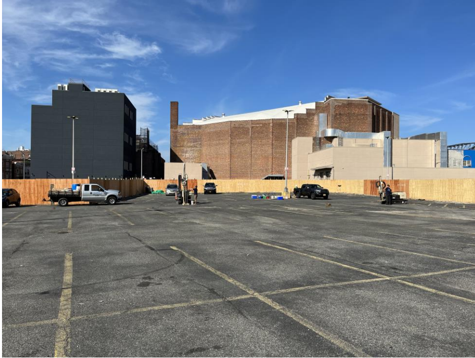
Photo 1: View of contractor advancing waste characterization borings, facing west.
