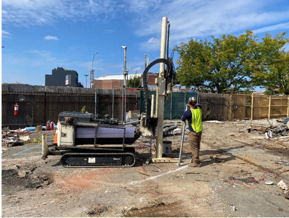
Photo 1: View of soil drilling activities, facing northwest.
