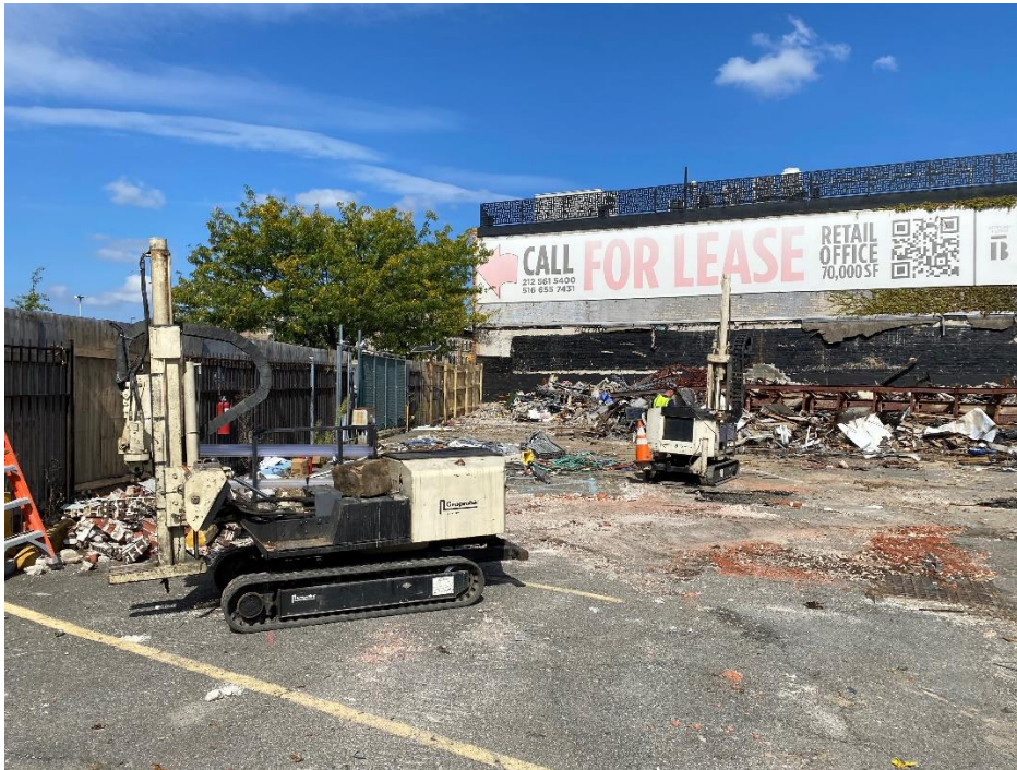
Photo 2: View of waste characterization soil boring activities, facing north.
