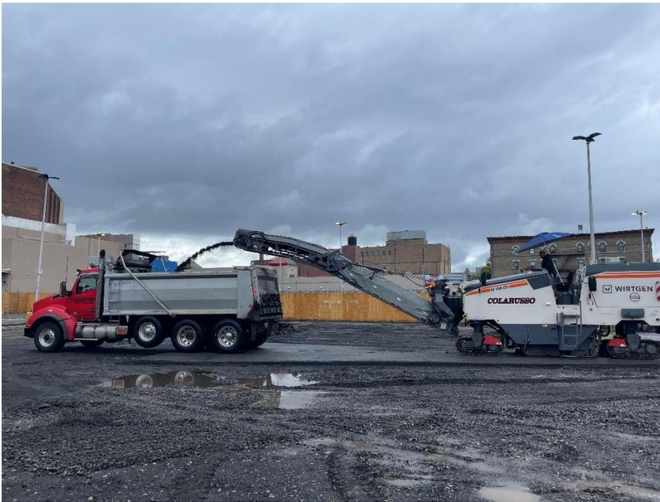
*Photo 2: View of asphalt stripping, facing north.*
