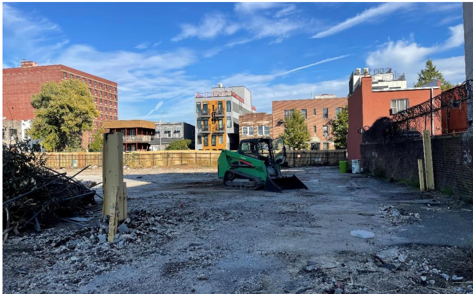
Photo 2: View of demo work in Lot 53, facing east.
