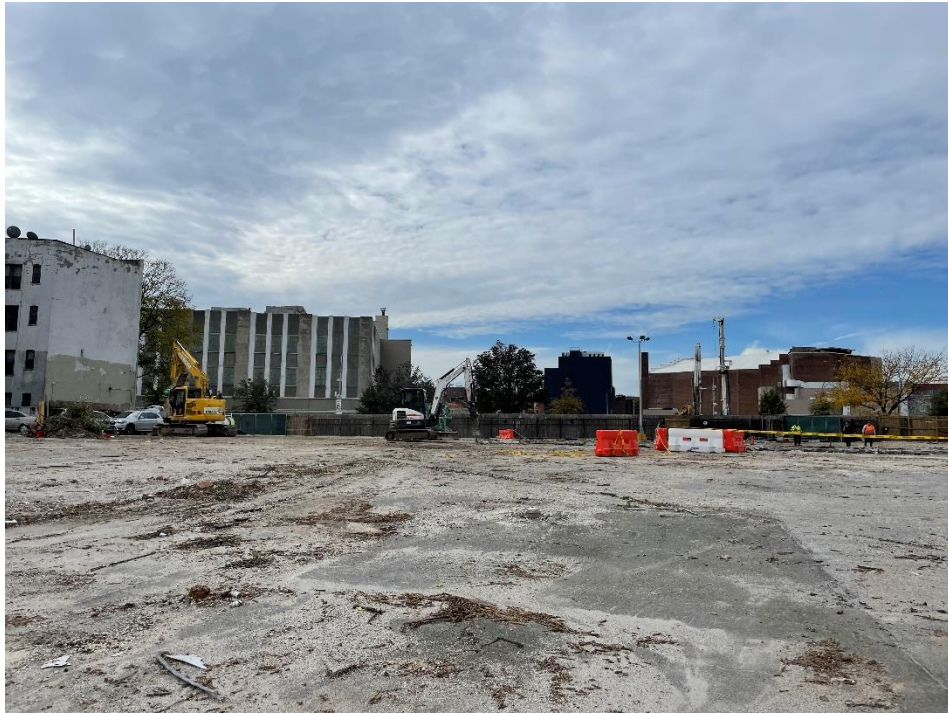
Photo 1: View of demo work in Lot 53, facing west.
