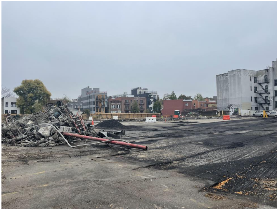
Photo 2: View of contractor conducting demo work of Lot 53, facing southeast.
