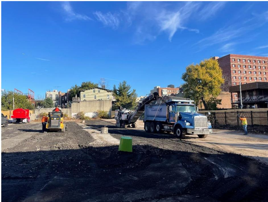
*Photo 2: View of contractor stripping asphalt of Lot 53, facing northeast.*
