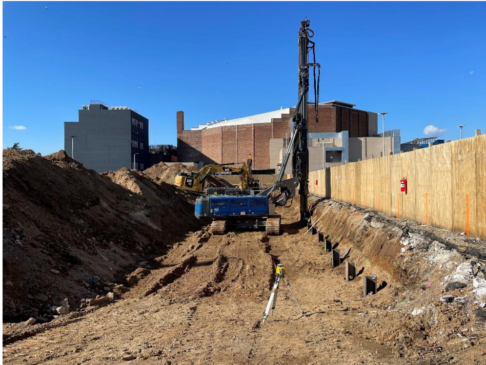
Photo 1: View of contractor installing H piles from lot 14, facing northwest.
