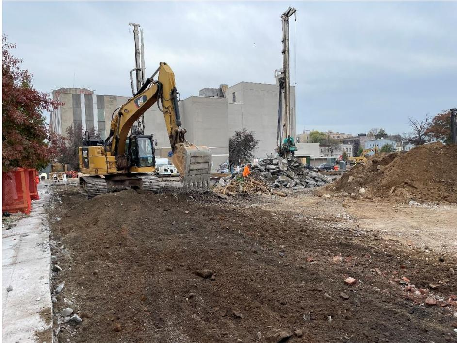
*Photo 1: View of excavation for SOE installation along the perimeter of Lot 14, facing south.*
