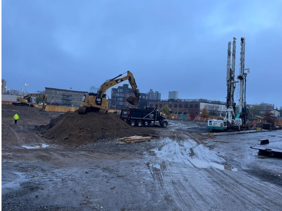
Photo 1: View of contractor loading soil in Lot 14, facing north.
