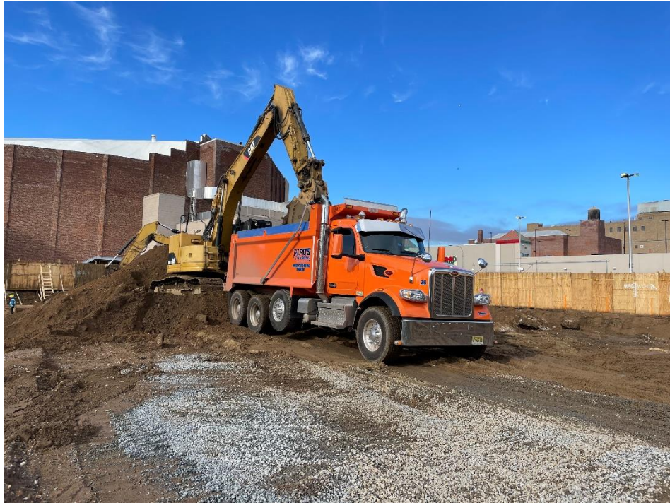
Photo 2: View of contractor loading soil on Lot 14, facing west.
