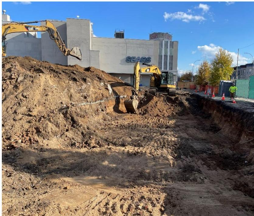
*Photo 2: View of excavation for SOE installation along the southern perimeter of lot 14, facing east.*
