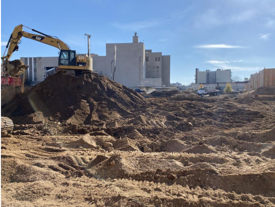
Photo 1: View of general site conditions of Lot 15, facing south.
